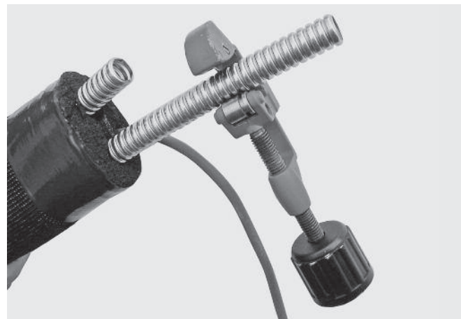
Fig. 3 Cutting to length using the pipe cutter
